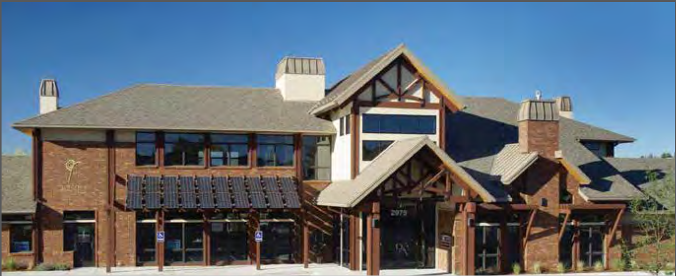
The south-facing front of this dental office in Loveland, Colorado demonstrates how awnings can be used to provide exterior shade. It also shows how the orientation of a building can lend itself to creative sustainable solutions, as seen in the solar panel awning.
