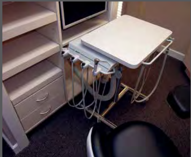
Flexible rear delivery serves both the doctor and assistant using a dental cart. To allow freedom of movement around the head of the patient chair, regardless of delivery type, the utility "umbilical" device tubing and foot control tubing/wiring must not be on or touch the surface of the floor.
