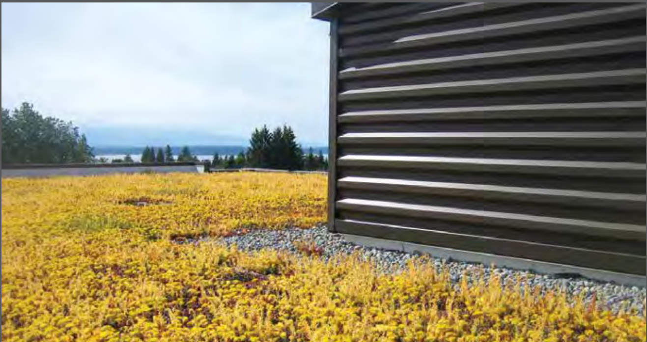
The green roof is a critical element to the project, creating a more energy efficient, environmentally beneficial and longer lasting roof assembly.
