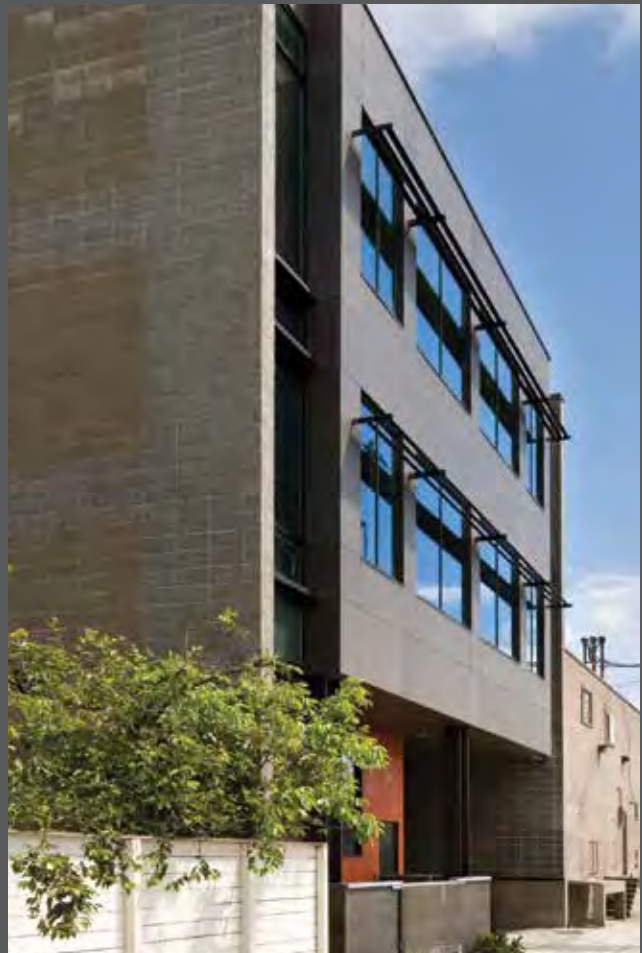
Sun shades help minimize heat gain and glare to maintain a comfortable interior environment.
