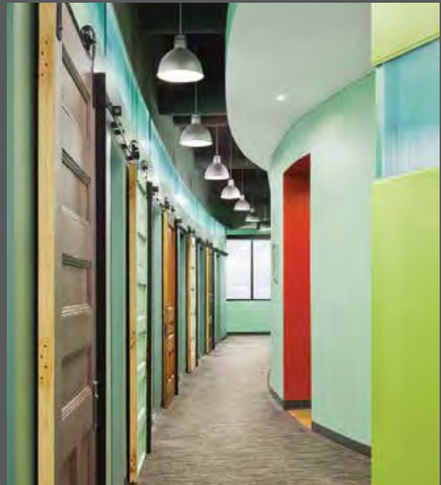
This sliding barn door uses salvaged doors and black-iron rail hardware for an eclectic feel.
