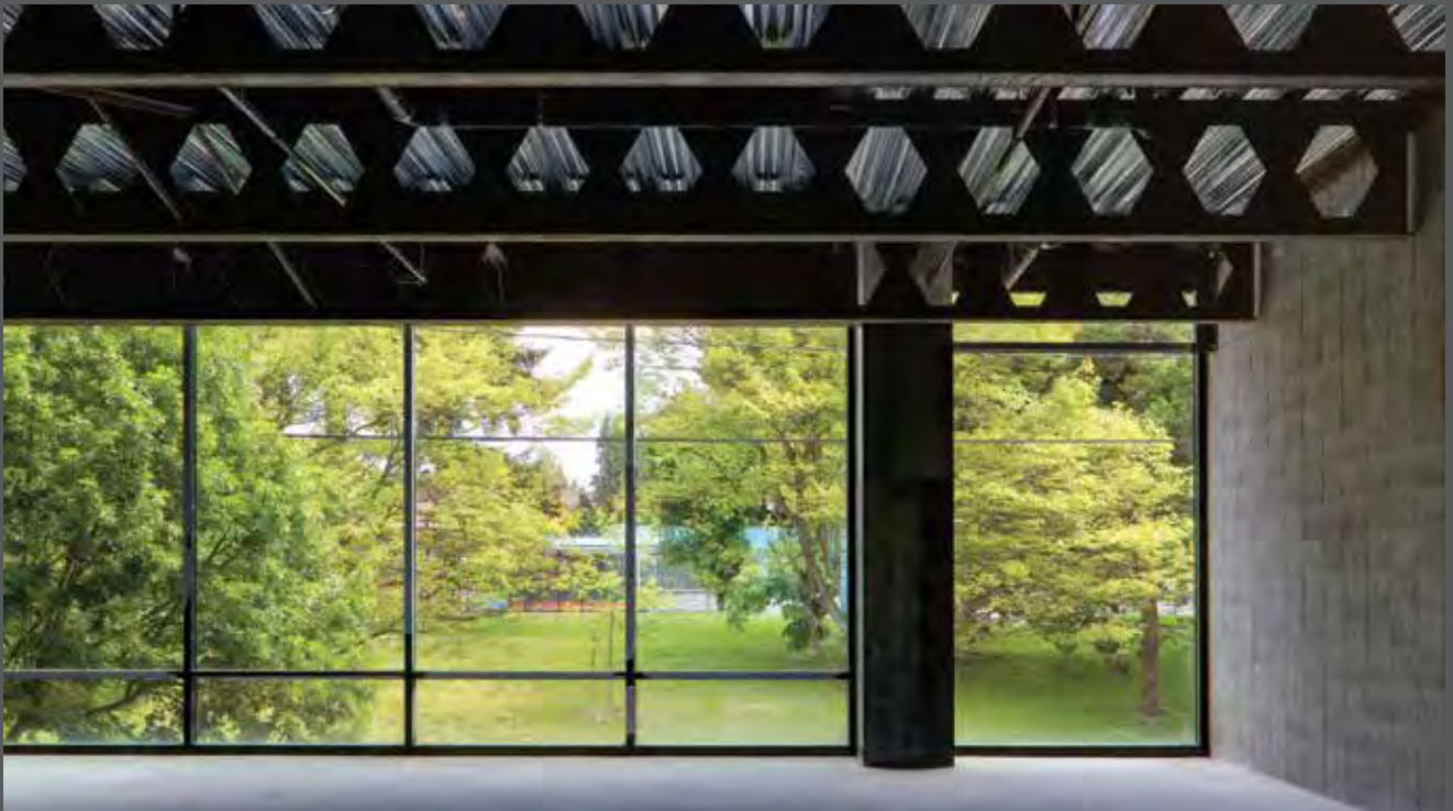
The interior floor plan was designed with minimal columns to provide flexible office space and maximize views of adjacent park.
